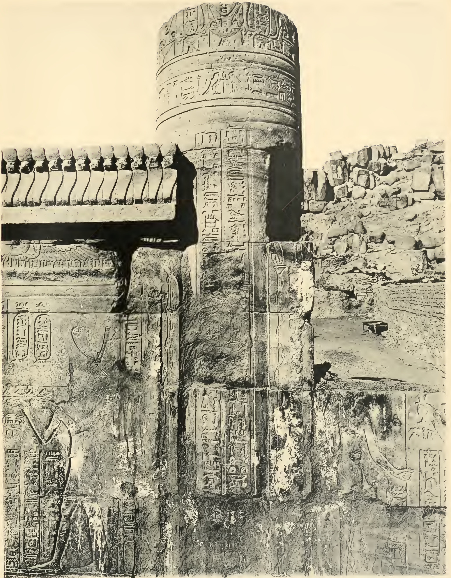
Outer Hall : East Face of Screen : Column 1.
