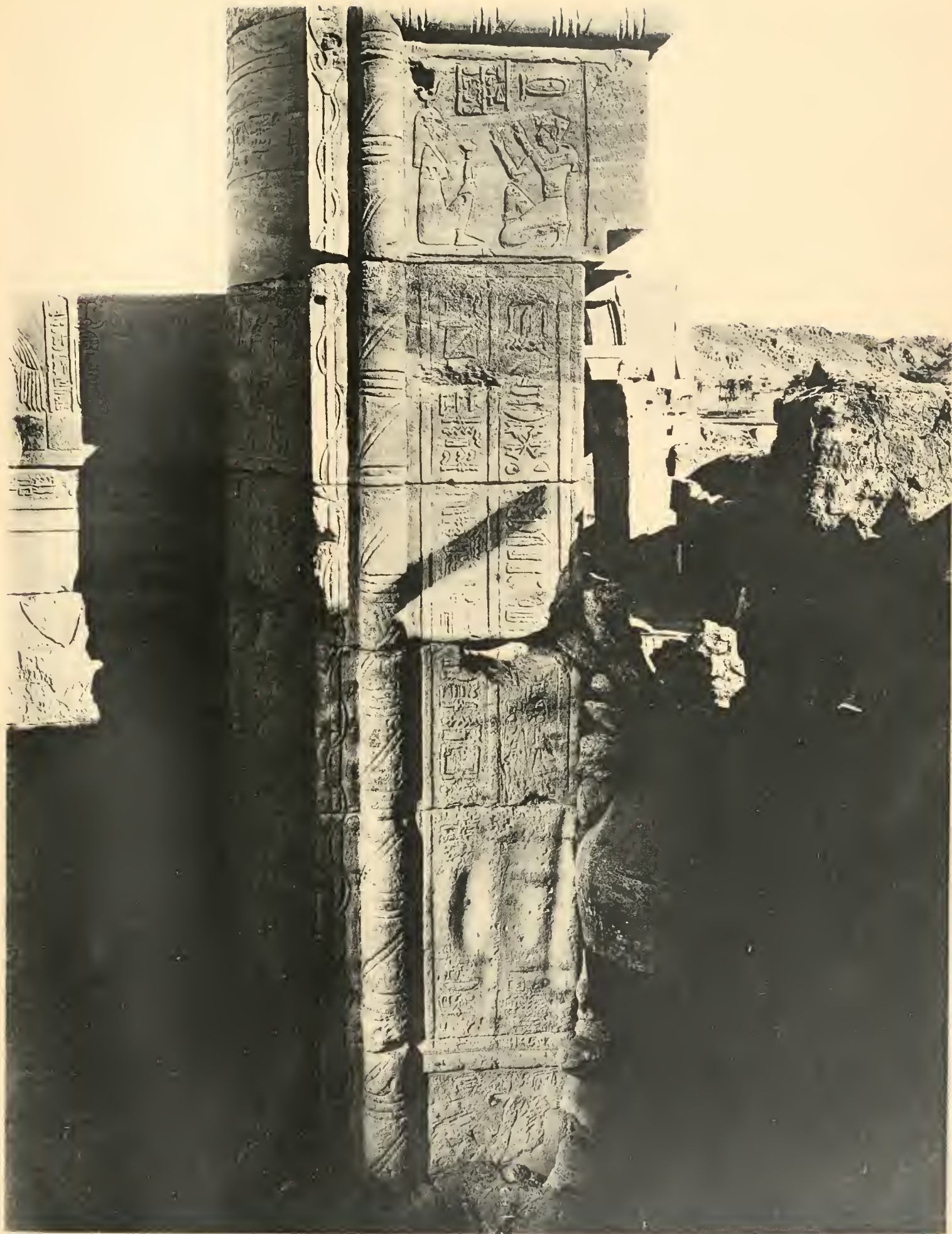
Outer Hall : Entrance : West Face : North Jamb.
