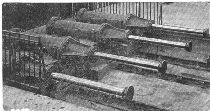
7 feet Hydraulic Buffer Stops at Waterloo Station for stopping 400 ton trains at 10 miles per hour.
