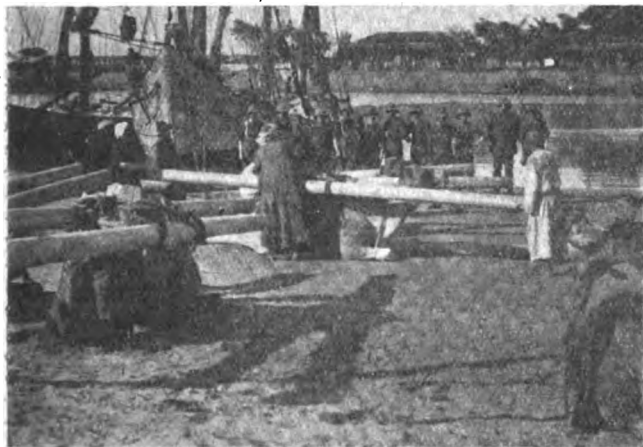
Pipes for pipe-line being unloaded from dhows at Kantara and put on to camels.
