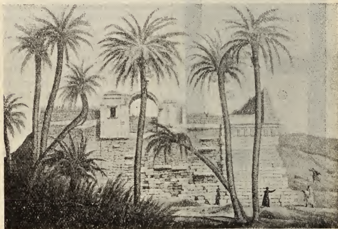
Remains of a building at Al-Qaşr. (From Cailliaud.)
