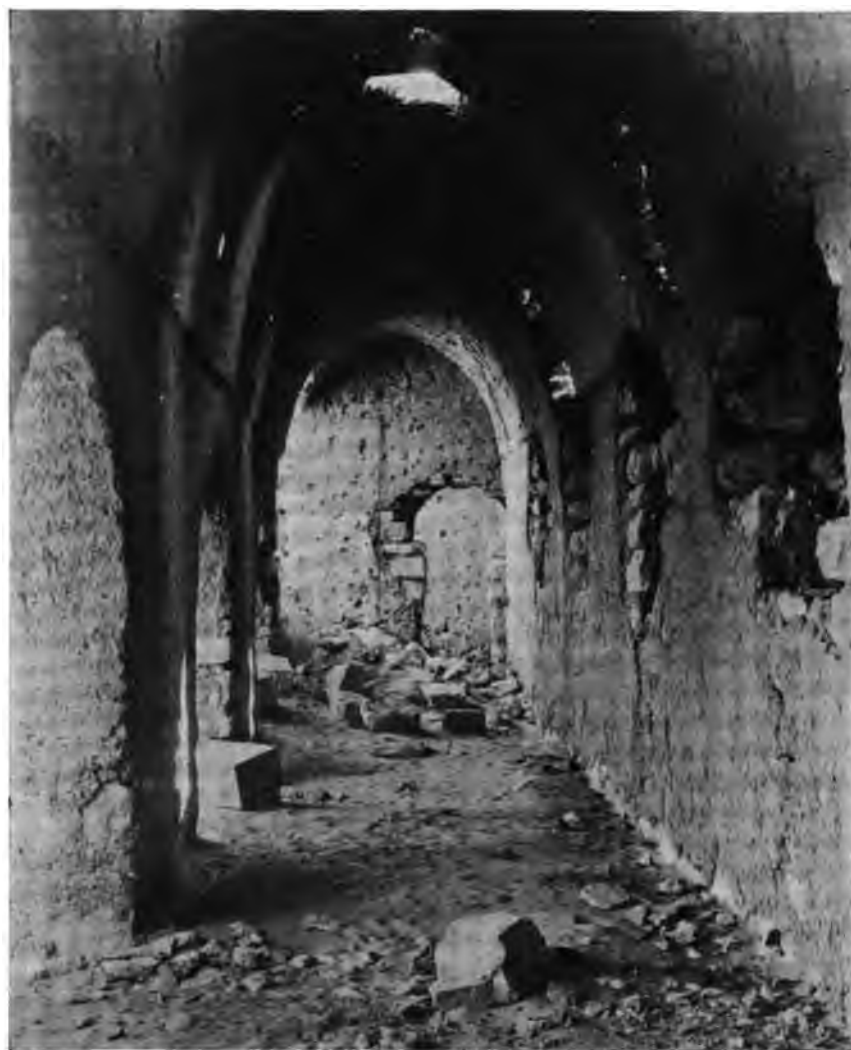
(b) The south aisle looking east.
