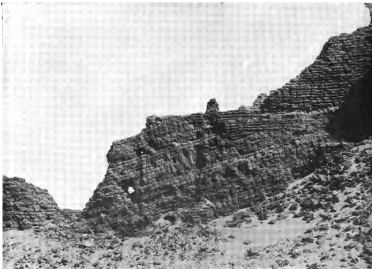
(b) The fortress wall, south side.
