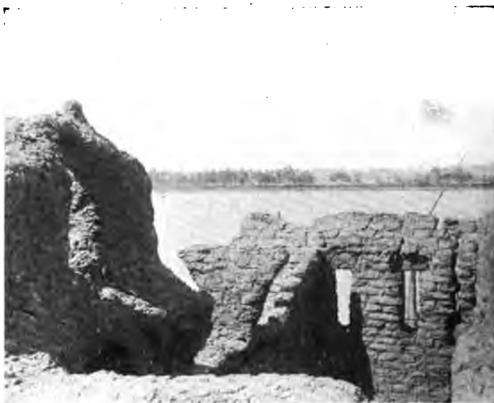
(b) View at roof level from northeast.
