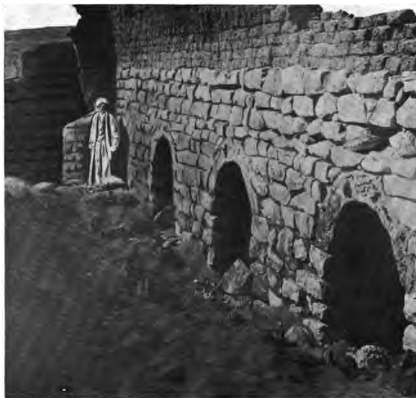
(a) Interior looking west, before excavation.
