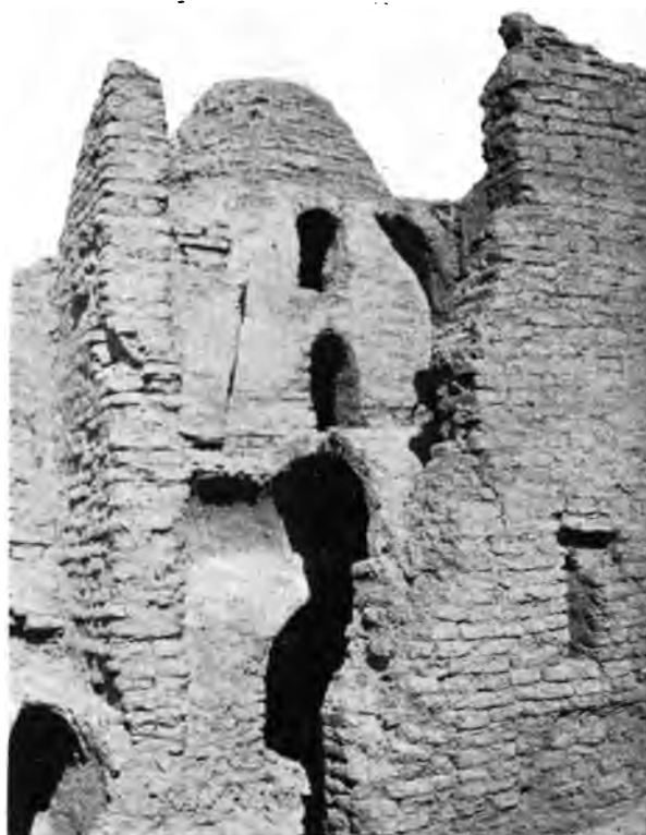
(b) View of dome from the south.
