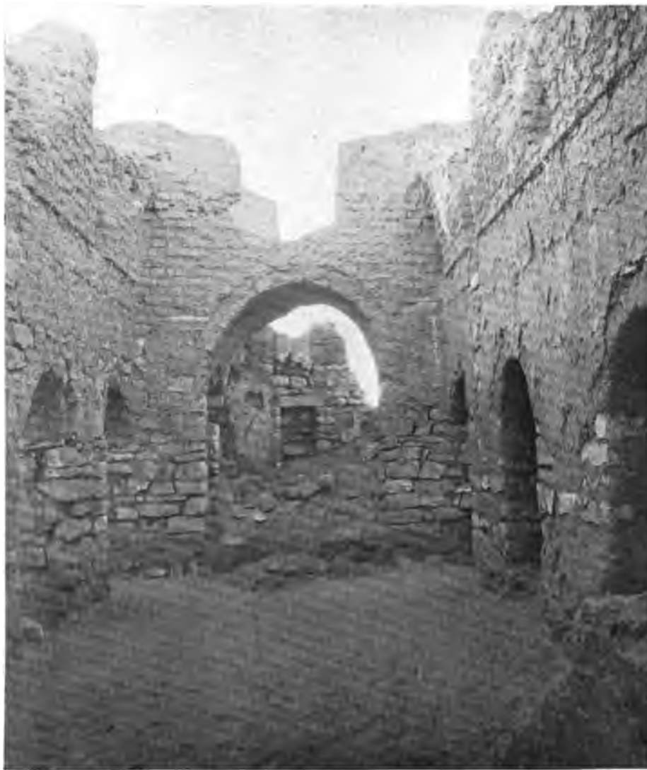
(c) Interior looking west.
