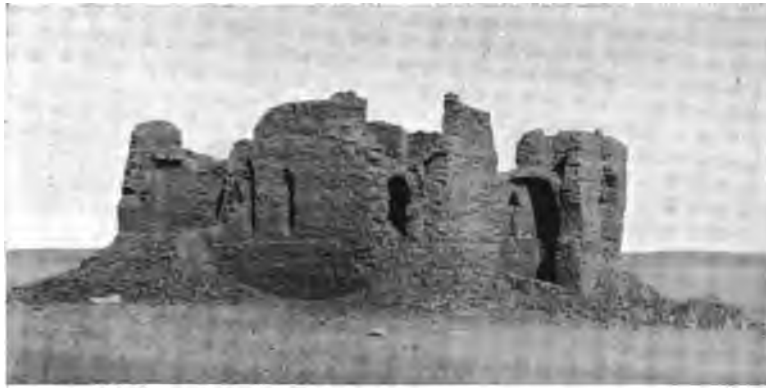
(a) View from southwest.
