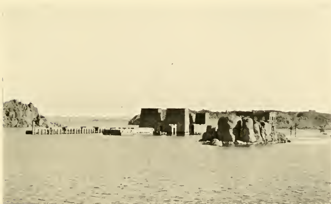
PHILAE, WITH THE ASSUAN DAM IN THE BACKGROUND
