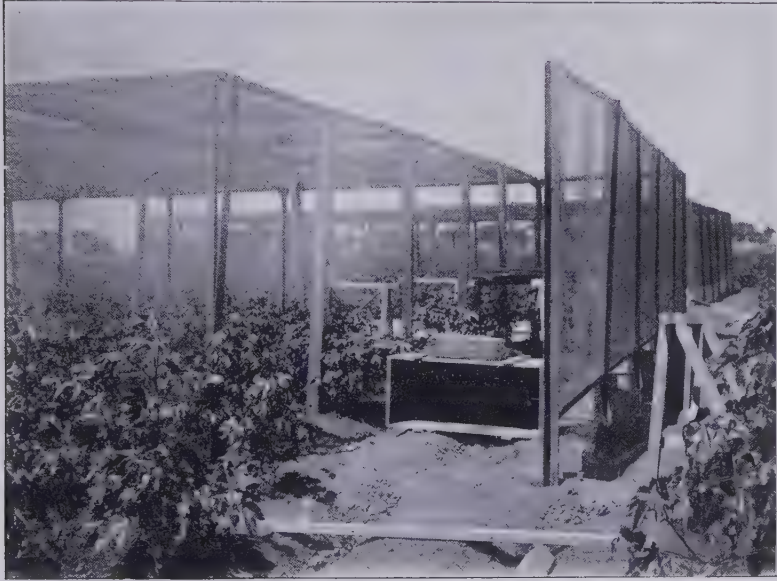
Bee-proof Cages. Showing "panel" construction on a sectional system. Note the transparency of three thicknesses of gauze as shown by the distant trees.
