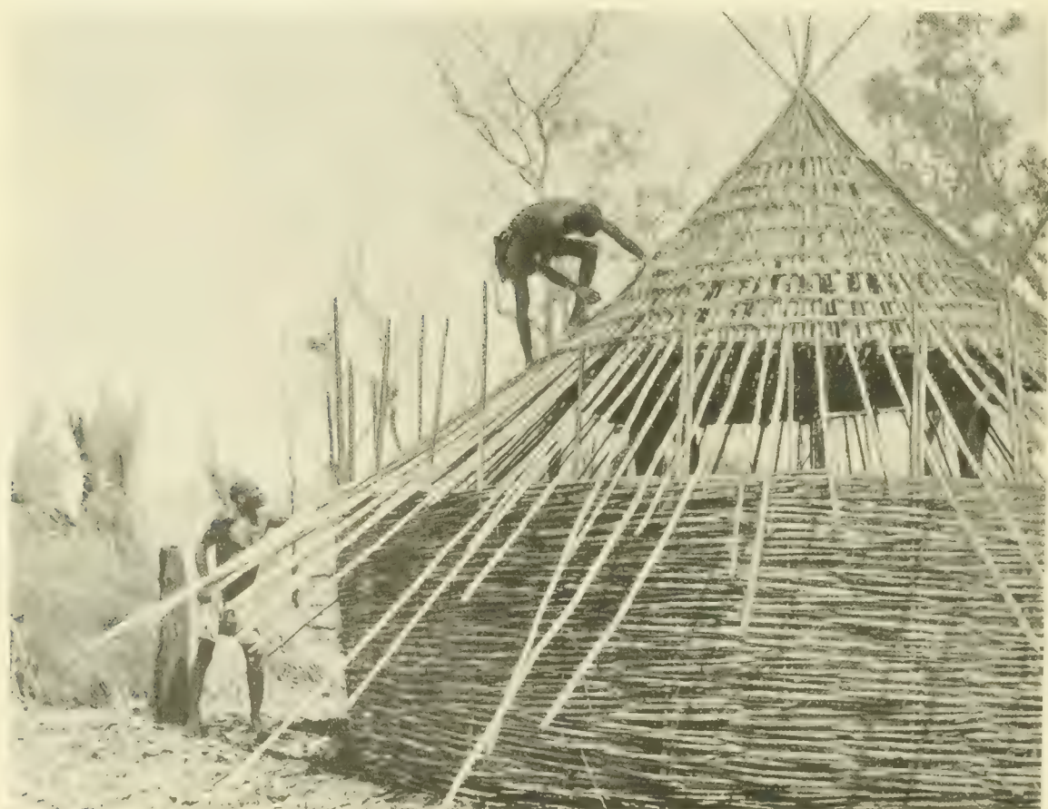
FIG. 50.—BURTAS BUILDING BAMBOO HUTS
