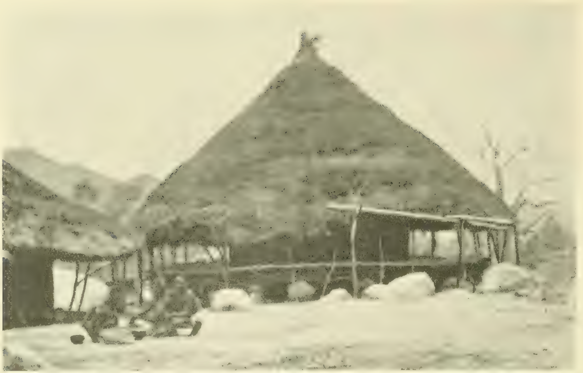
FIG. 153.—OMDA'S HUT, JEBEL KEILI. BUILT IN STONE TO KEEP OUT WHITE ANTS
