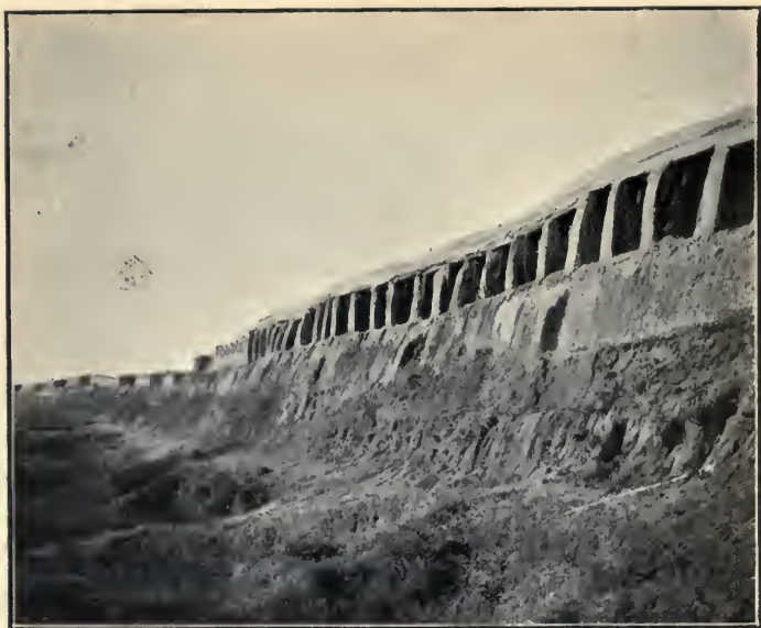
The Great Wall of Kano
