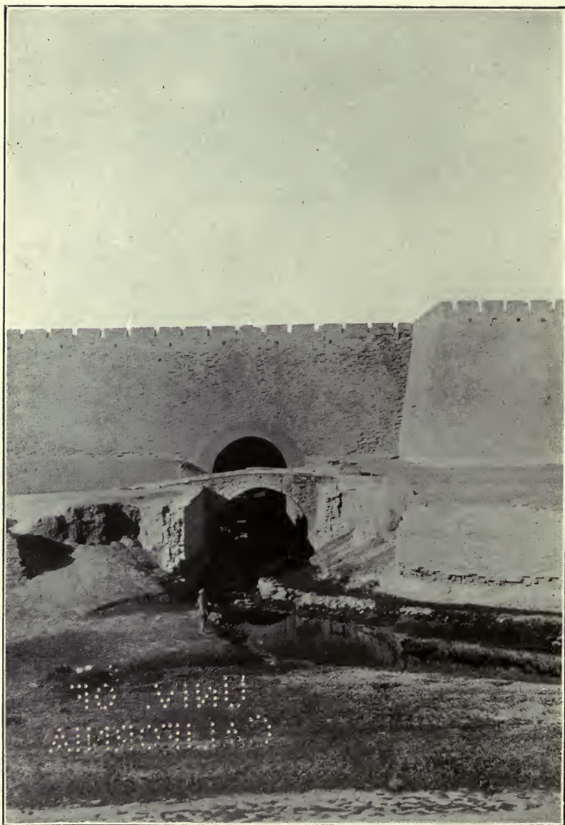
SLUICE GATE WHERE THE BRITISH ENTERED.
