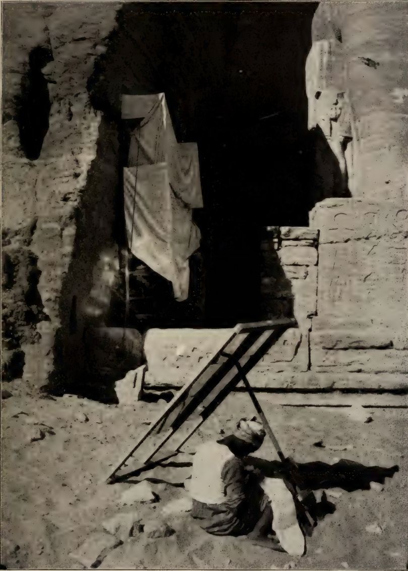
FIG. 4.—Method of Shading and Illuminating from a Reflector Erected at One Side. The sunshine on the inscription before the copyist on the scaffolding comes from the reflector beside the native in the foreground. The inscription, covered with canvas to exclude the excess of light, is the stela at Abu Simbel recording Ramses II's marriage to a Hittite princess.
