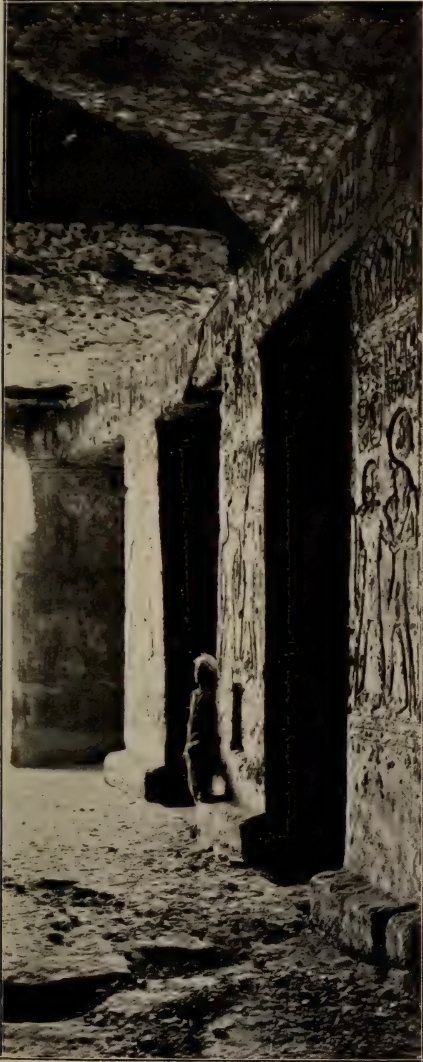
FIG. 27.—Hall of the Temple of Derr, showing Bend in Architrave.
