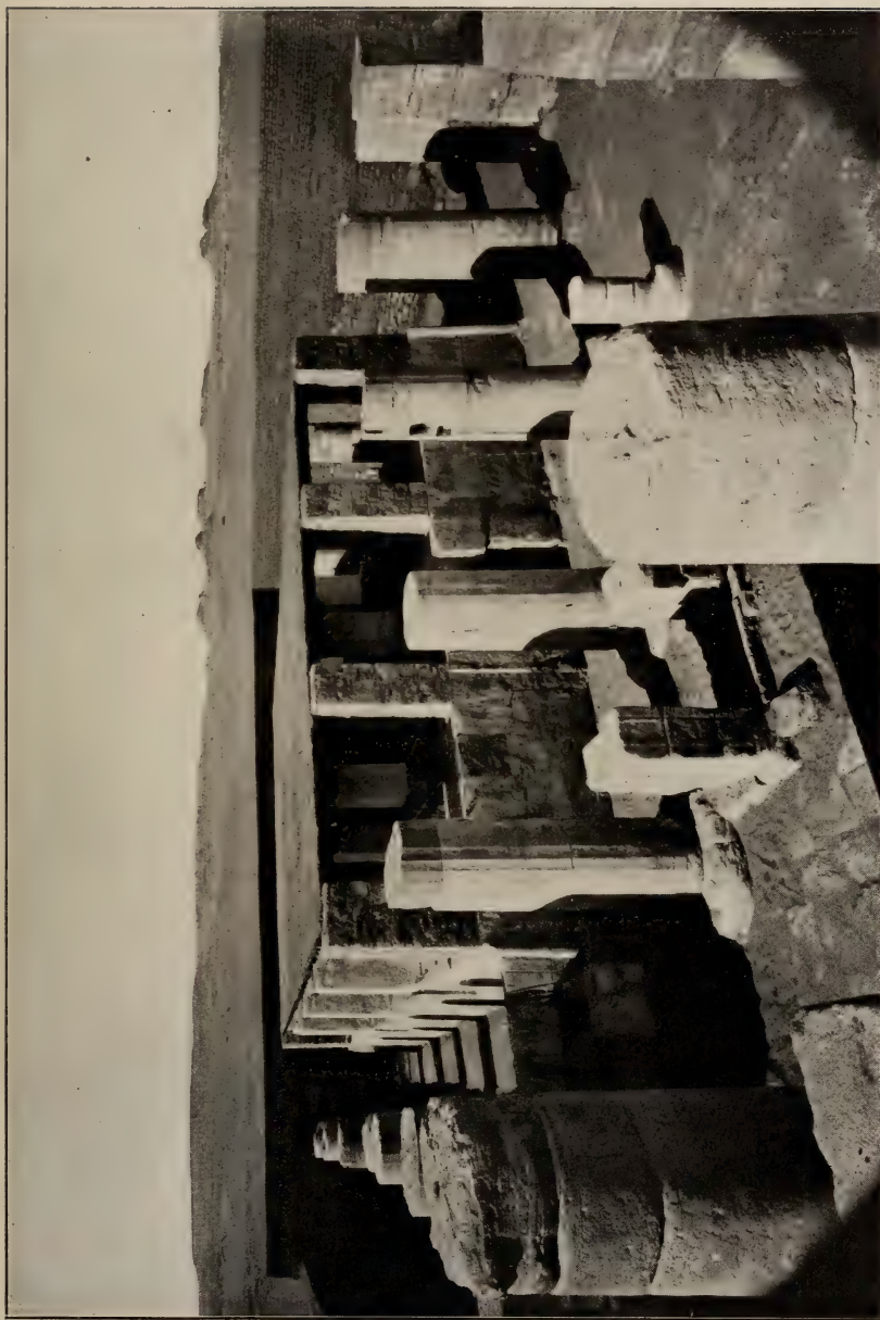
FIG. 5.—Temple of Thutmose III and Hatshepsut at Halfa. The roof, the square pillars bearing it, and the surrounding wall are modern works for the protection of the temple, erected by Mr. Scott-Moncrieff, of the British Museum.
