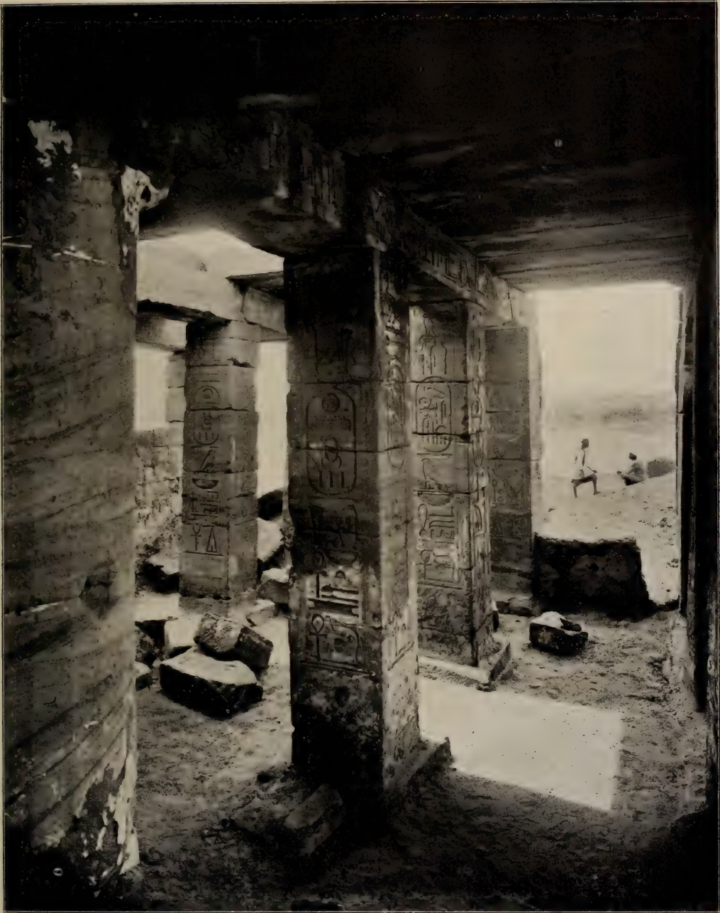
FIG. 32.—First Hall of the Temple of Amada after Excavation. Viewed from r (on plan), including from pillar 4 (at right) to 1 (at left) and 12 (at right) to 15 (at left). The depth of the excavation may be seen by comparing the cartouches or royal ovals on the square pillars in Fig. 30 with those on the same pillars above (Fig. 32).
